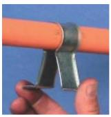
Squeeze strap back around pipe. (NOTE: Pipe must be allowed to move freely)
