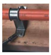
3. Fasten the strap to the wood surface using the two screws provided. (#10 x 1 hex washer head unslotted, self-tapping.)
