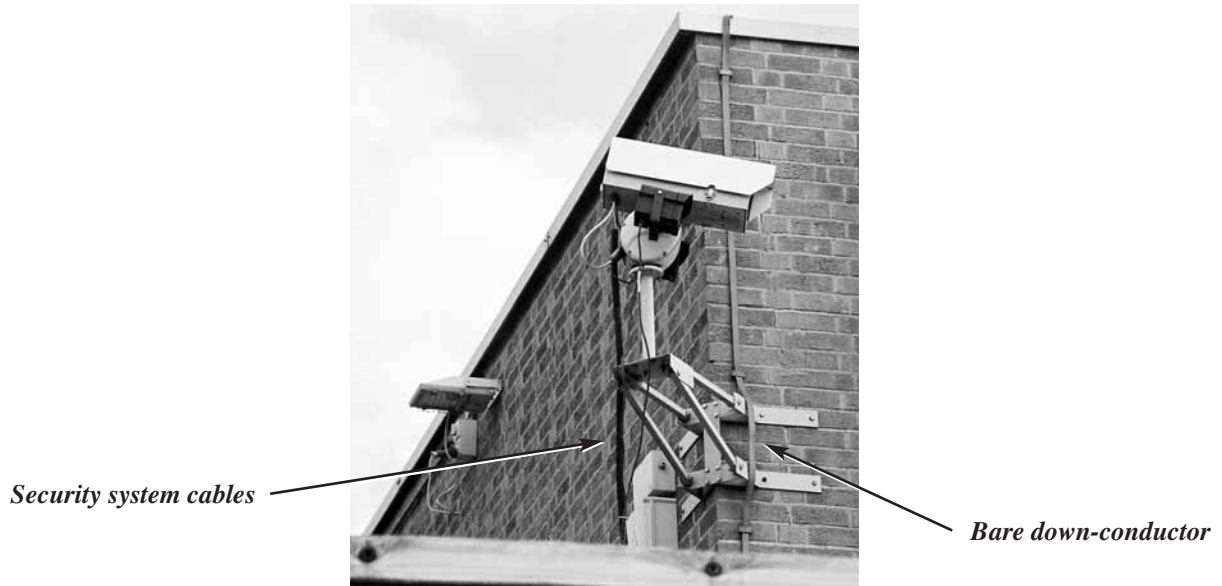
Figure 2. Conventional down-conductor separation distance problem.
