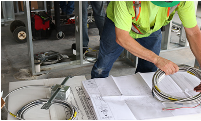
STEP 1 Perform the layout using the provided installation drawings and stickers
