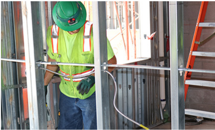
STEP 3 Pull the cable
